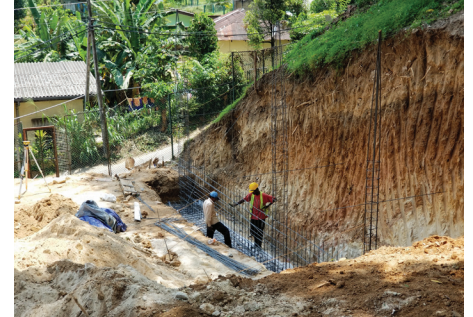
Commerce block Grid 7 concrete wall base Reinforcements and column starters
