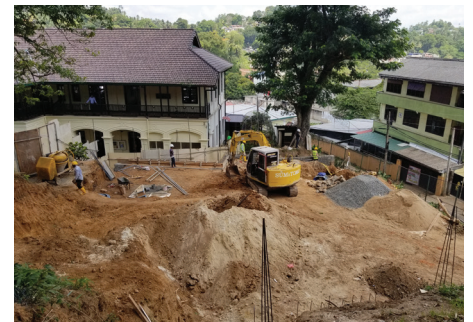
Back filling and excavation for column bases in progress
