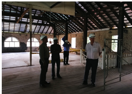
Alison House second floor perimeter wall plastering
