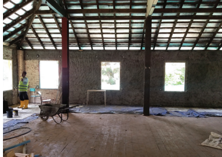
Alison House second floor perimeter wall plastering
