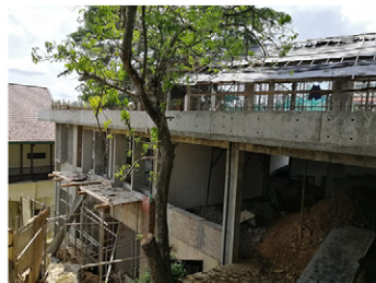
External view of the new Classroom Block
