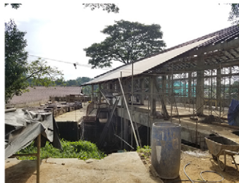
Roof and open terrace of the new Classroom Block
