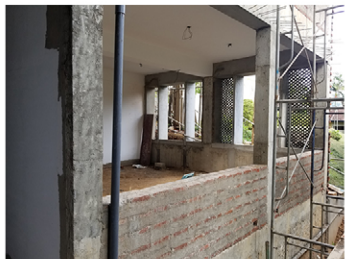
External view of the new Classroom Block Ground Floor
