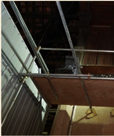
Images above: Scaffolding fixtures during the restoration and cleaning process of the Chapel's Chancel
