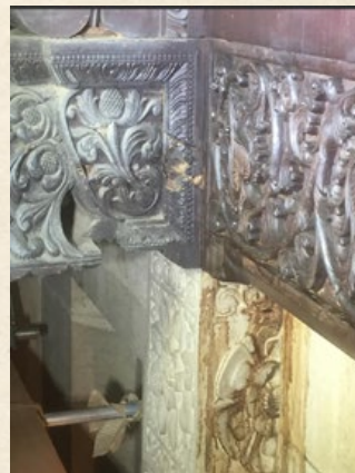
Images left: Damaged wooden 'pekadas' in the chancel - due to rainwater leakage, damage by termites, and dust gathering.
