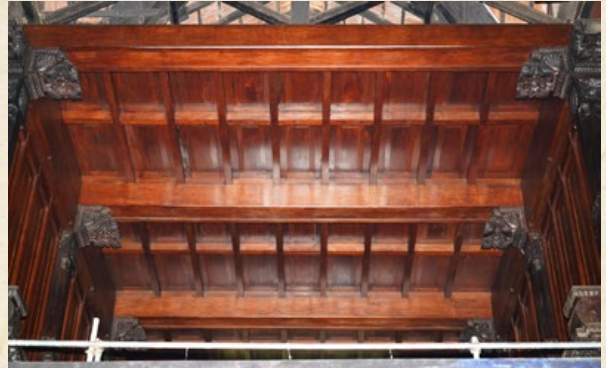
Images left: Damaged wooden 'pekadas' in the chancel - due to rainwater leakage, damage by termites, and dust gathering.
