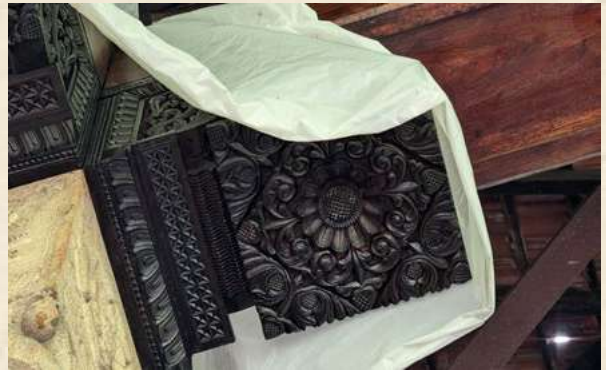
Images left: Damaged wooden artwork - due to rainwater leakage, damage by termites, and dust gathering.
